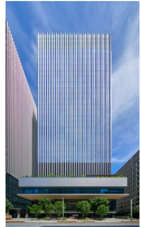
Exterior of the new office building
